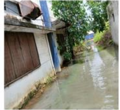
Water Logging in the Factory
