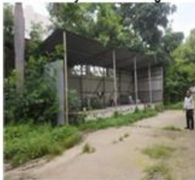
Material Loading Platform
